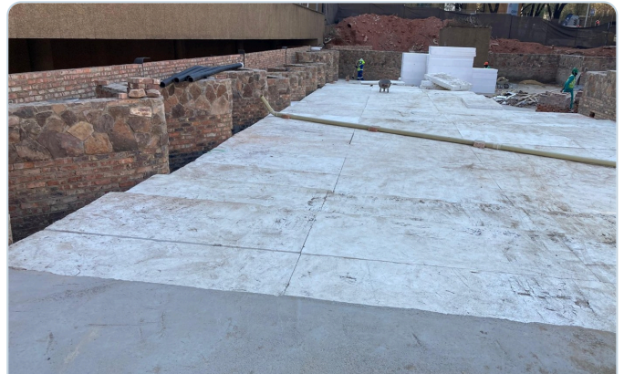
Completed works — RC slab cast over the fill, ready for the structure above.
