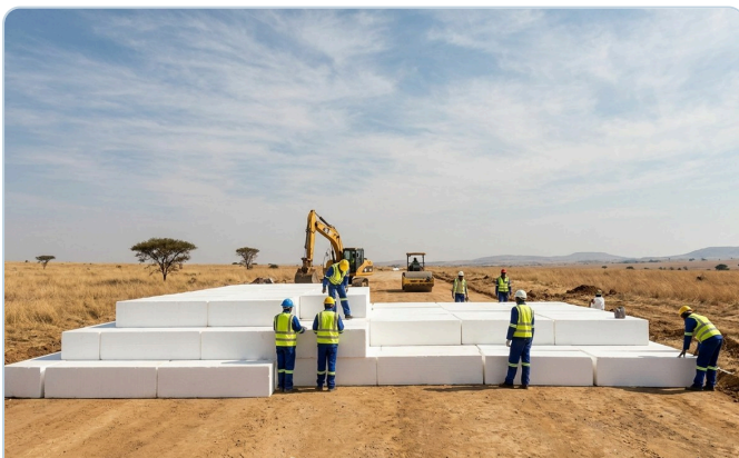
Road embankment — lightweight fill over soft ground.
