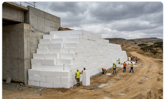
Bridge approach — geofill against the abutment.
