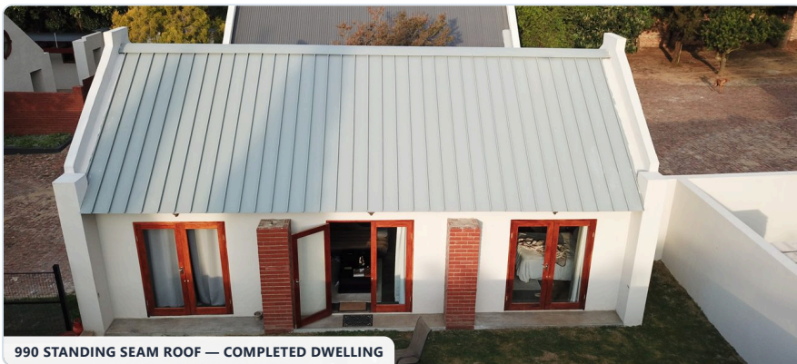
990 STANDING SEAM ROOF — COMPLETED DWELLING
