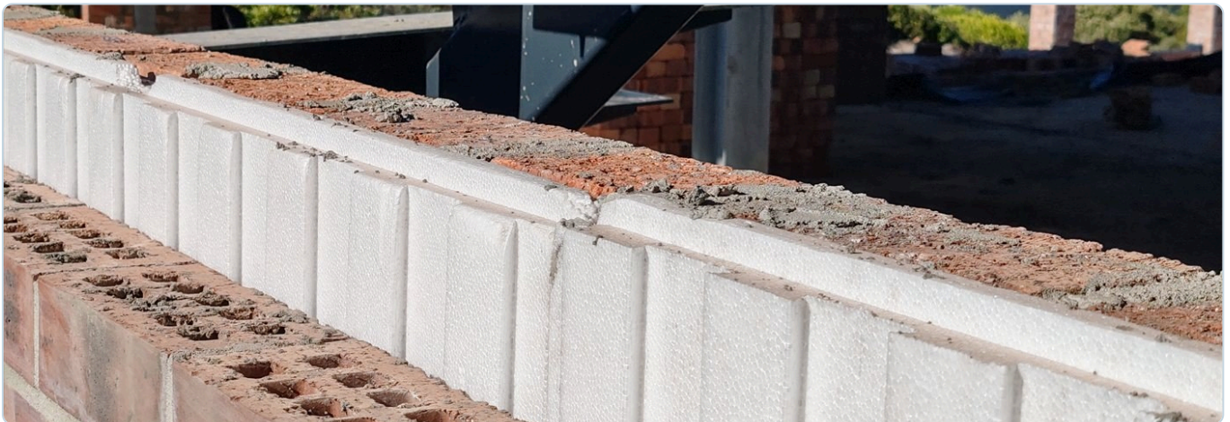
Fire-retardant EPS cavity-wall boards built into a coastal face-brick wall (2025) — one of four verified bulk-board application families.
