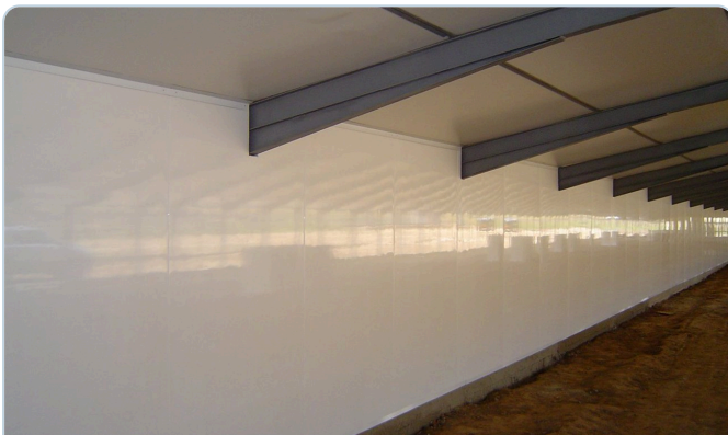
Interior — long white insulated wall-to-ceiling lining.
