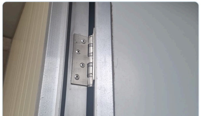
Door hinge — stainless butt hinge on the aluminium jamb.
