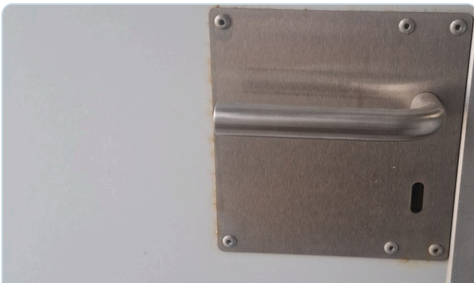
Door furniture — stainless lever and lock plate on a panel-door skin.
