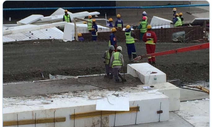
Placement — blocks positioned over the reinforced base and worked into the fill by hand.
