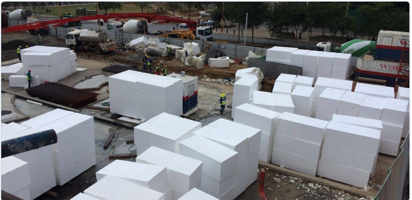
Technopol EPS geofoam blocks on site — lightweight structural fill, delivered in large blocks and cut to shape.
