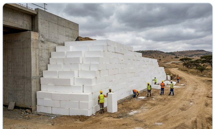
Bridge approach — geofill against the abutment.
