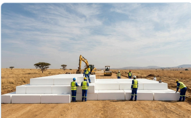
Road embankment — lightweight fill over soft ground.
