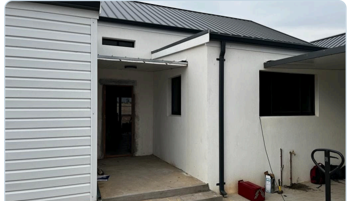
Finished house entrance — wall cladding meeting a standing-seam roof and a plastered wall; the metal face is the finish.
