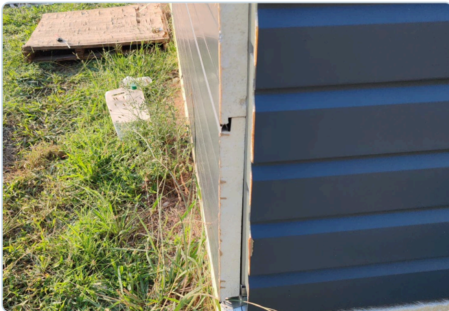
Wall corner (Our Shack project) — the steel weatherboard cladding meets an exposed return, with the external EPS insulation edge and galvanised base flashing visible at the trim.
