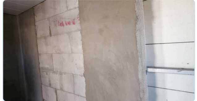
Left: the composite block — white EPS core between lightweight-concrete skins, with tongue-and-groove interlock. Right: the wall build-up on site — bare blocks, then mesh-reinforced LiteCore Plast render.
