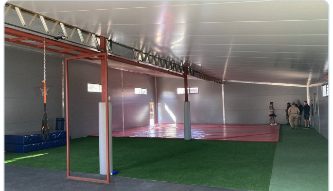
Long-span commercial — panels as walls and roof over lattice trusses in a sports hall.
