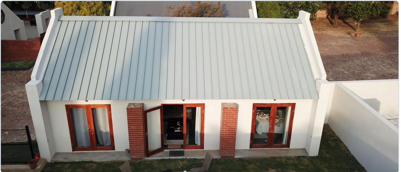
A completed LiteSpan 990 Standing Seam roof (Winn Kyalami) — a single panel forms structure, insulation, weatherproofing and the finished ceiling.
