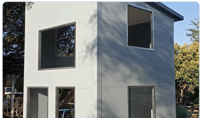
Clean elevations — horizontal wall-panel joints and a mono-pitch panel roof.
