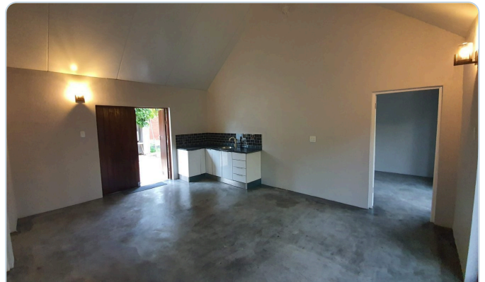
Roof is the ceiling — the white panel underside as the finished pitched ceiling, no separate lining.
