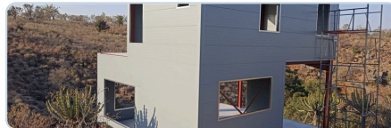
Walls & cladding — T&G panels
