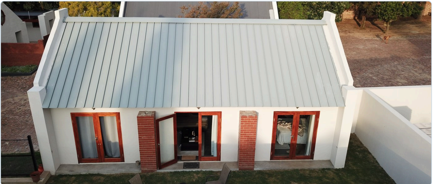
LiteSpan 990 standing-seam roof panels installed on a South African project — factory-laminated FRCel EPS core between coated-steel skins.
